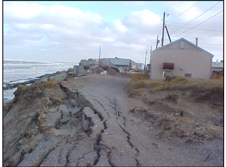
Photo 9: Erosion near Shishmaref homes. (Credit: Brice Eningowuk )
